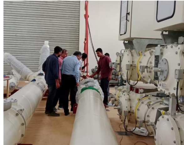
Consultants observed the GIS installation
