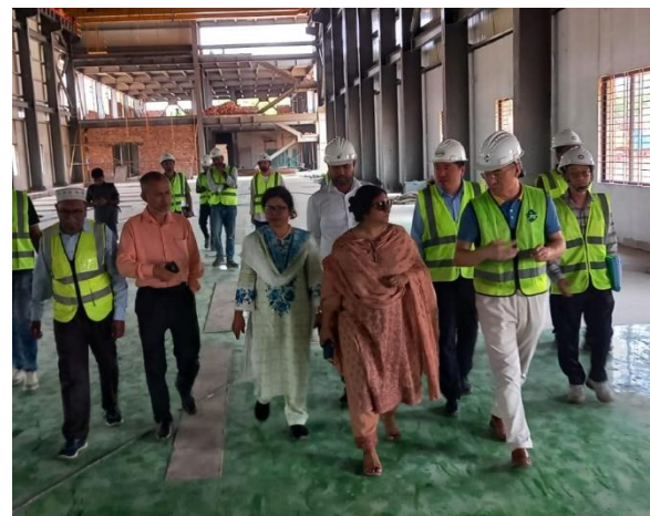
Power Ministry officials & Consultants visit Korheraat 400/230kV GIS Substation
