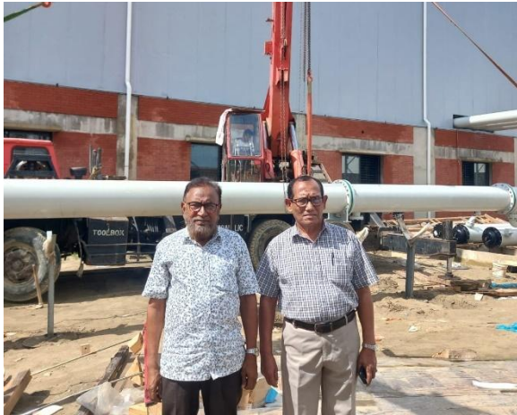
Chairman & Civil Consultant visit Korheraat 400/230kV GIS Substation
