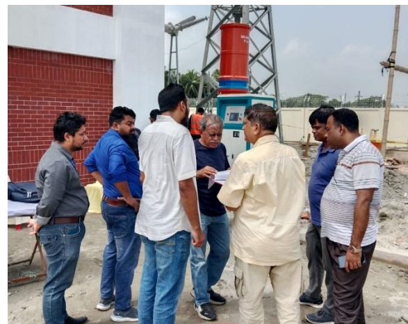
Consultants instruct the EPC team for High voltage test
