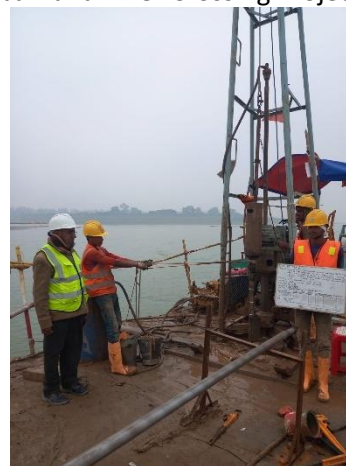
Soil exploration works at new BH No.4DR7. The last depth of this BH is 6.0m. The last depth of BH No.4DR8 is 109.5m, and the last depth of BH No.4DR1 is 45m
