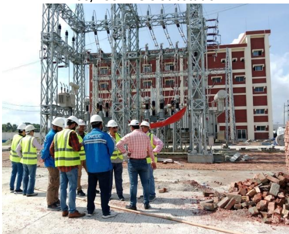
Consultants visit the Substation
